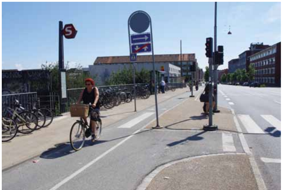
A short section of a two-way cycle track and a signalized cyclist crossing makes the Nørrebro cycle route continuous and cohesive.
