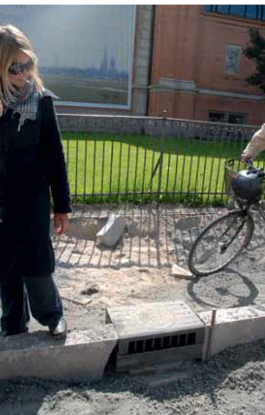
When cycle tracks are very narrow, rain water gullies built into the kerb remove rough spots making the cycle track more bikeable.
