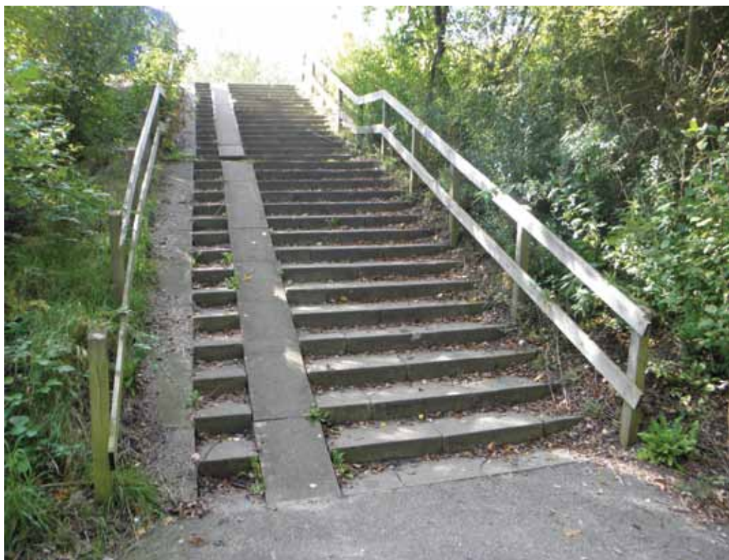
Combined bike and pram ramp.
