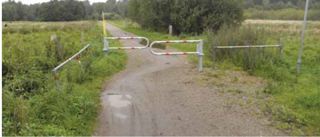
Barriers are set up to reduce moped speeds.
