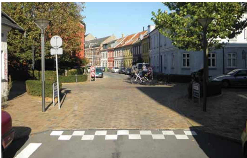
The crossing is raised to pavement level.
