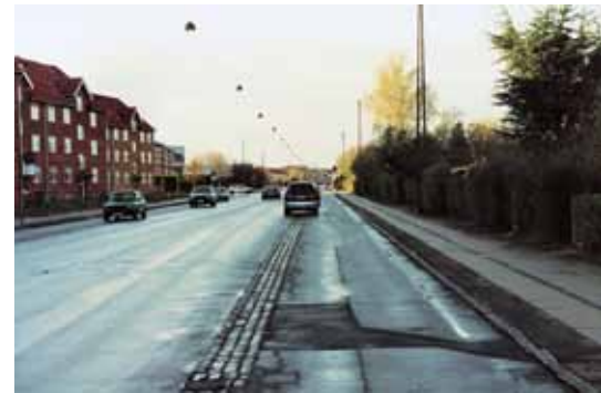
Segregation of road and cycle track.
