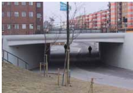
This Malmö cycle tunnel provides excellent visibility thereby enhancing cyclist's sense of security.
