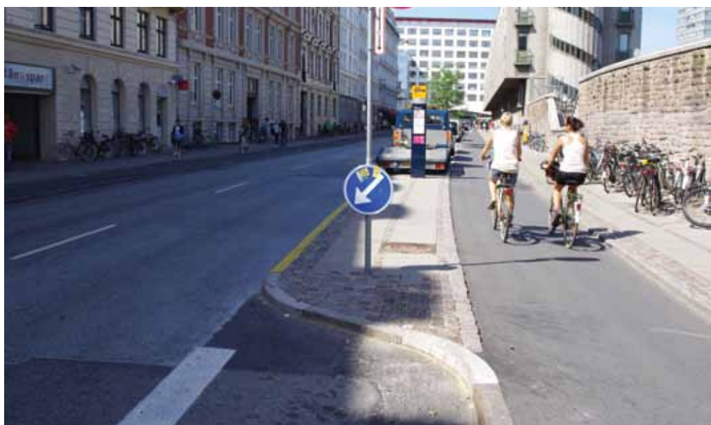
Bus nub (kerb extension) where the waiting area between the cycle track and the bus takes space from the cross profile. Car traffic – but not cycle traffic – has to wait while the bus stops at the bus stop.
