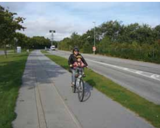
New cycle tracks along Koktvedvej in Frederikshavn. The cycle track and pavement are clearly segregated by a beveled kerb. This facilitates cleaning and winter maintenance of cycle tracks and pavements.
