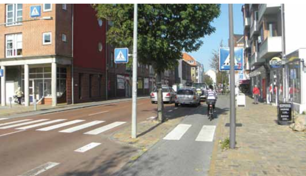
Safe crossing for pedestrians across the cycle track.
