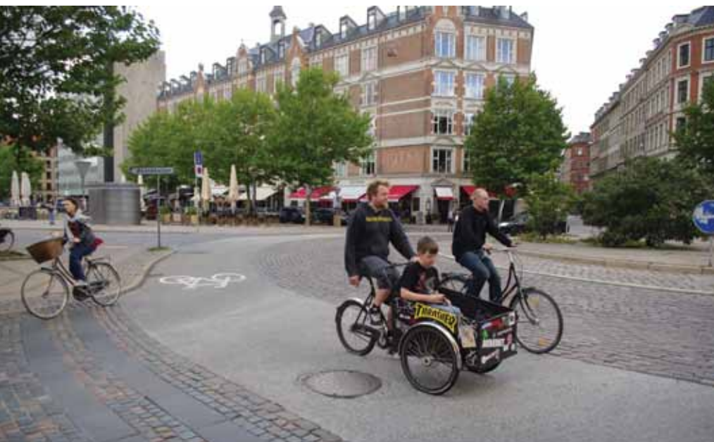
Traffic calmed roundabout with tarmacked cycle lane all the way around. Halmtorvet, Copenhagen.
