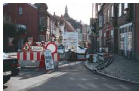
One way of improving cycling facilities is during utility construction.
