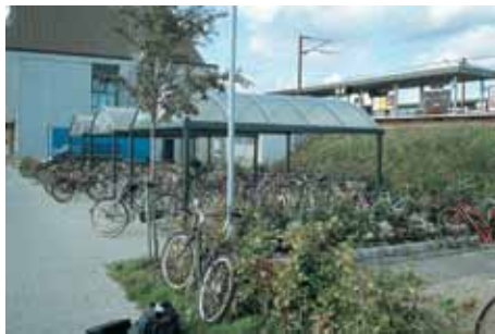
Covered bicycle parking facility at railway station
