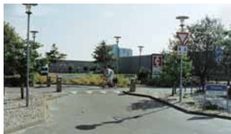
The cycle path crosses the road on a raised surface, and motorists have to give way to cyclists.
