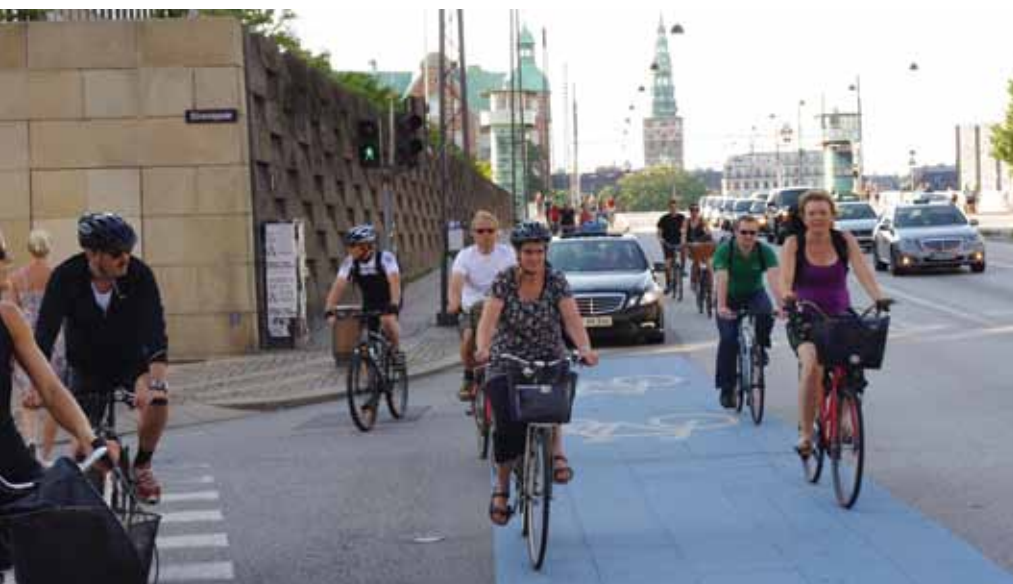
When the cycle track incline means that cyclists ride faster than normal the cycle track is shortened in the interests of cyclist safety. Knippelsbro bridge, Copenhagen.
