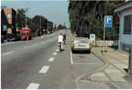
The parking bays here are too narrow. A car door is 0.9 m wide.
