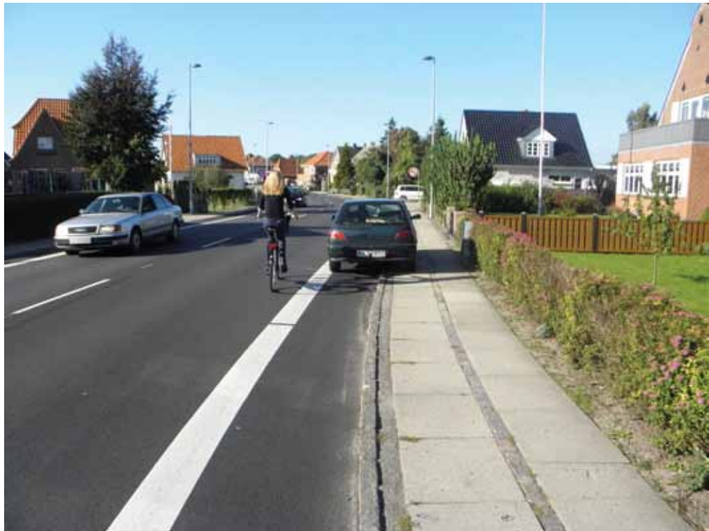
Parking on the cycle lane can put cyclists in a dangerous position.
