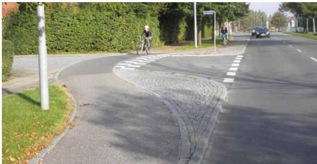
Set-back cycle track. The bend means that cyclists can't bike through the intersection faster than 20 km/h; motor vehicles have a waiting area on the outer edge of the cycle track.
