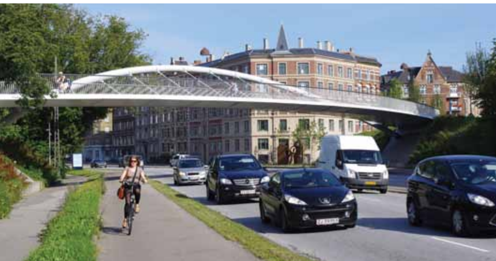
Åbuen. A bridge was the only feasible solution here as the alternative was a traffic signal which would significantly reduce motor vehicle capacity on this approach road. An underpass was not an option either since a stream runs under the road. The bridge links the municipalities of Copenhagen and Frederiksberg.
