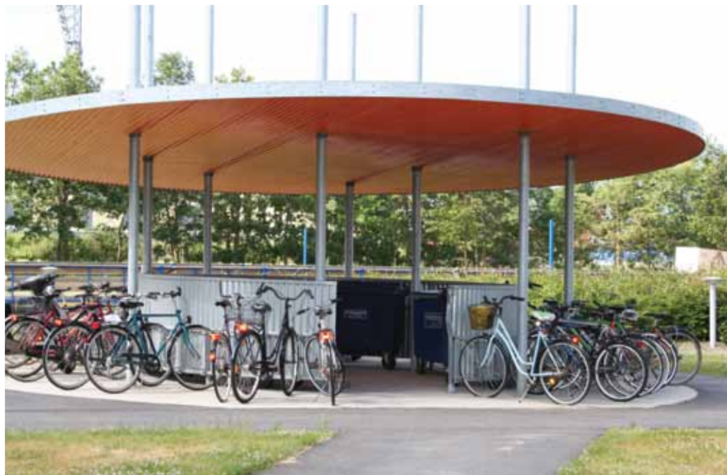
Covered bicycle parking facility at Viborg student residence combined with a rubbish disposal facility.
