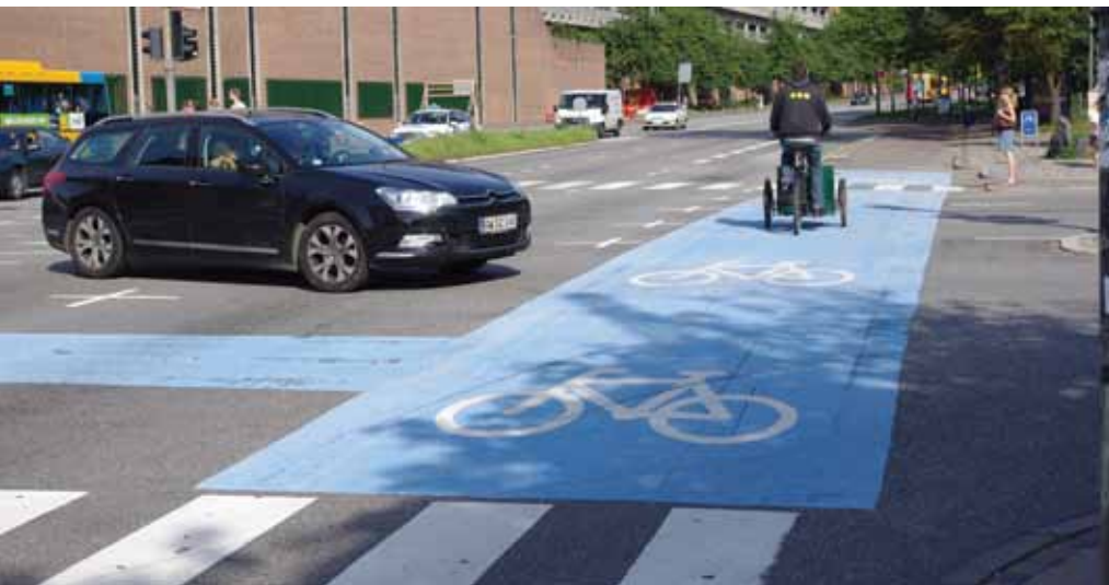
Internal road safety considerations in the City of Copenhagen tend toward using up to 2 blue cycle crossings per intersection, based on a concrete assessment of the individual situation. Tagensvej.
